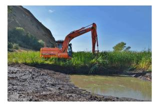
Asymmetrically excavated pond profile providing both depth (right) and gentle gradients (left).
